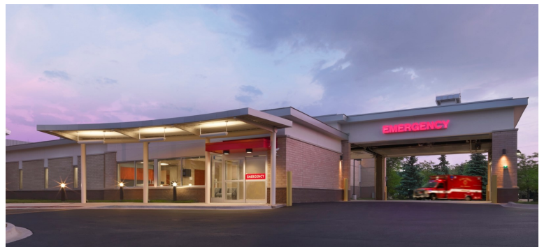
Vista Freestanding Emergency Room 1050 Red Oak Lane • Lindenhurst
