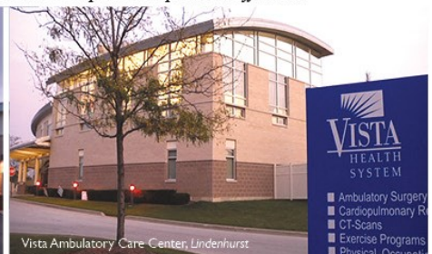
Vista Ambulatory Care Center, Lindenhurst
